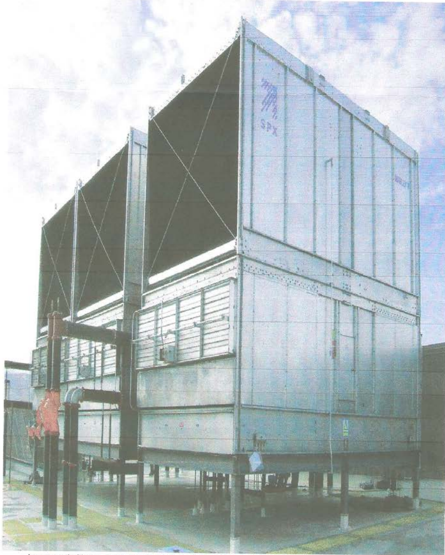
Figure 6.11 Indicative image of wet cell cooling towers
